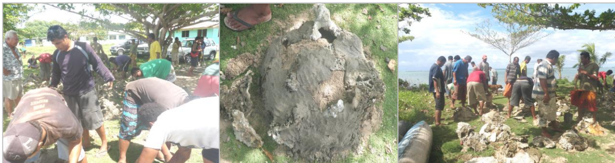
Village communities engaged in fish house construction work
