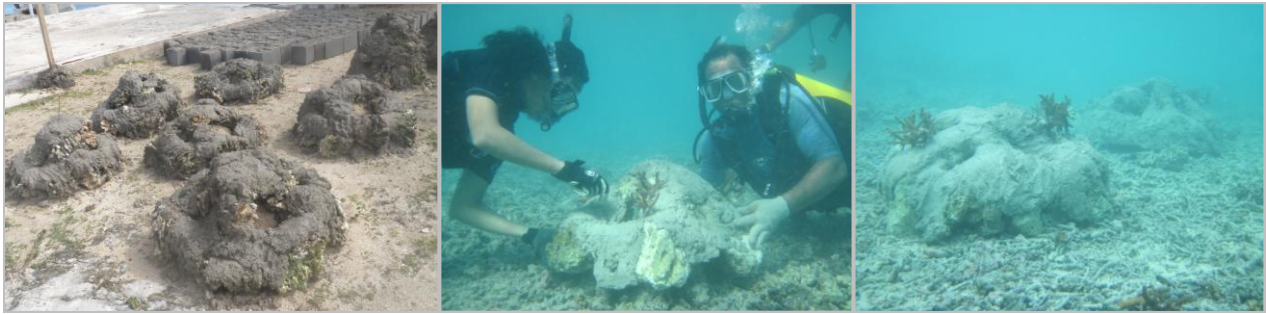
Artificial fish houses constructed
